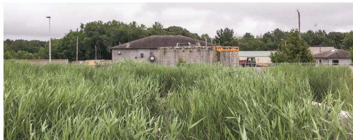
In 2015, the Mora Wastewater Treatment Facility received Clean Water Funds to construct upgrades that reduced phosphorus discharge to the Snake River by 74 percent.
