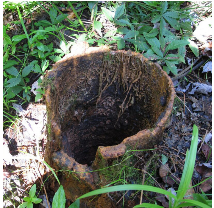
Figure 50. Abandoned wells pose a risk to groundwater.
