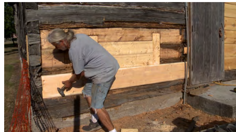
Local contractor Roy Schwartz replaces rotten log facings.
