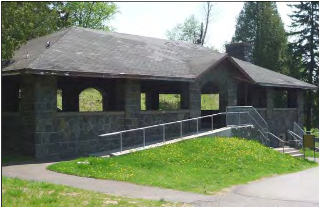
WPA Pavilion Before Renovations
