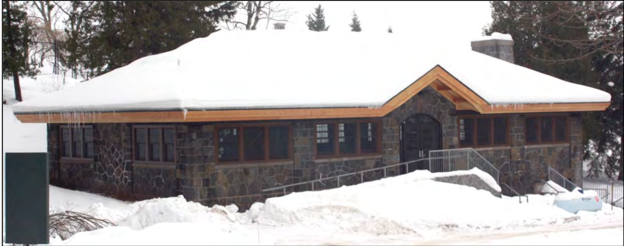
WPA Pavilion After Renovations
