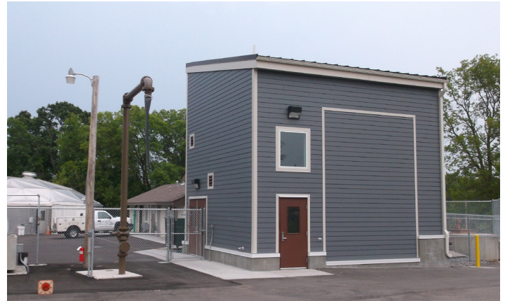
The Rockford Wastewater Treatment Facility built a chemical feed building as part of its work to reduce phosphorus discharge into the Crow River.
