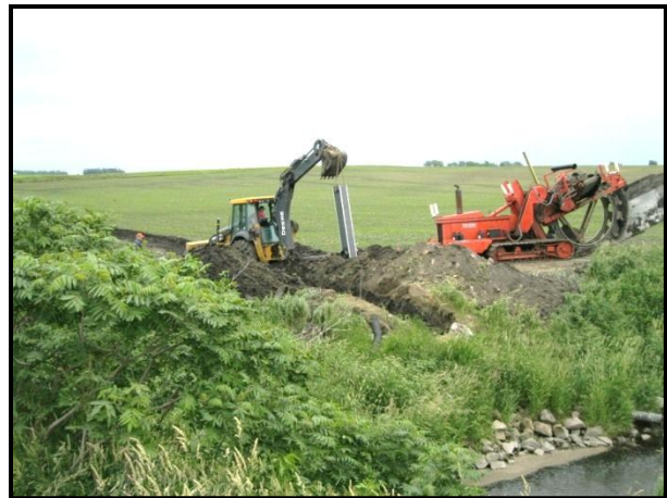
Figure 3.25: Installation of Agri Drain control structure at BE2, June 2011. Agri Drain provides access point for subsurface tile monitoring.
